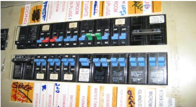
Main hydro panel is well labeled. Panel is full, and expansion would require a pony panel installation.
